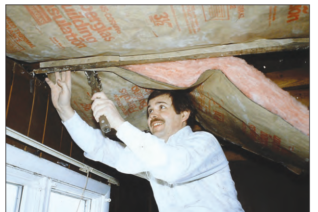
Art Thompson installs insulation in the new rehearsal space.
