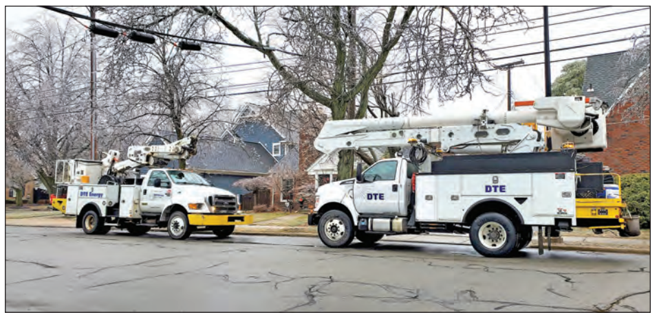
DTE Energy workers make repairs along Grosse Pointe Boulevard.
