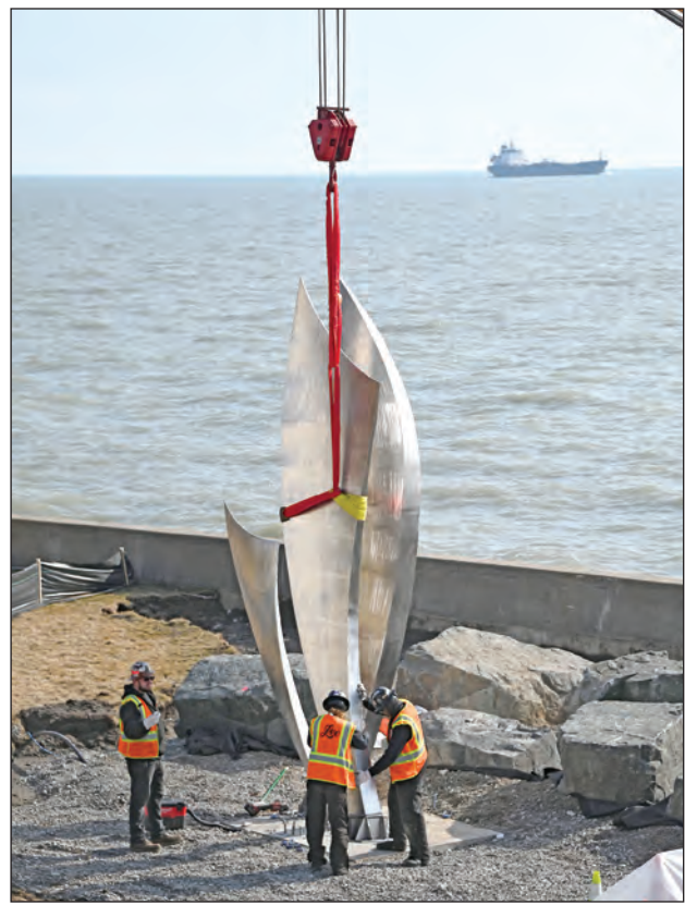
Left, the crew maneuvers the stainless steel piece by inch until it sits properly over the mounting bolts designed by the artist.
