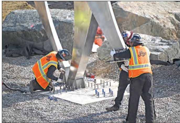
Left, the crew maneuvers the stainless steel piece by inch until it sits properly over the mounting bolts designed by the artist.
