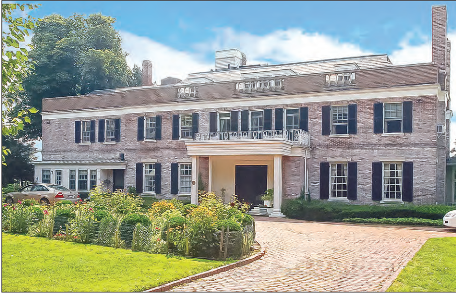
A front view of 2 Woodland Place.
