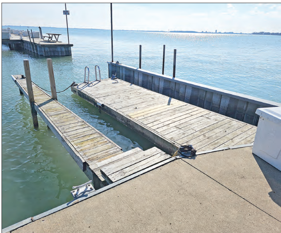
New plans will improve accessibility at the kayak launch, which currently can prove challenging to kayakers.
