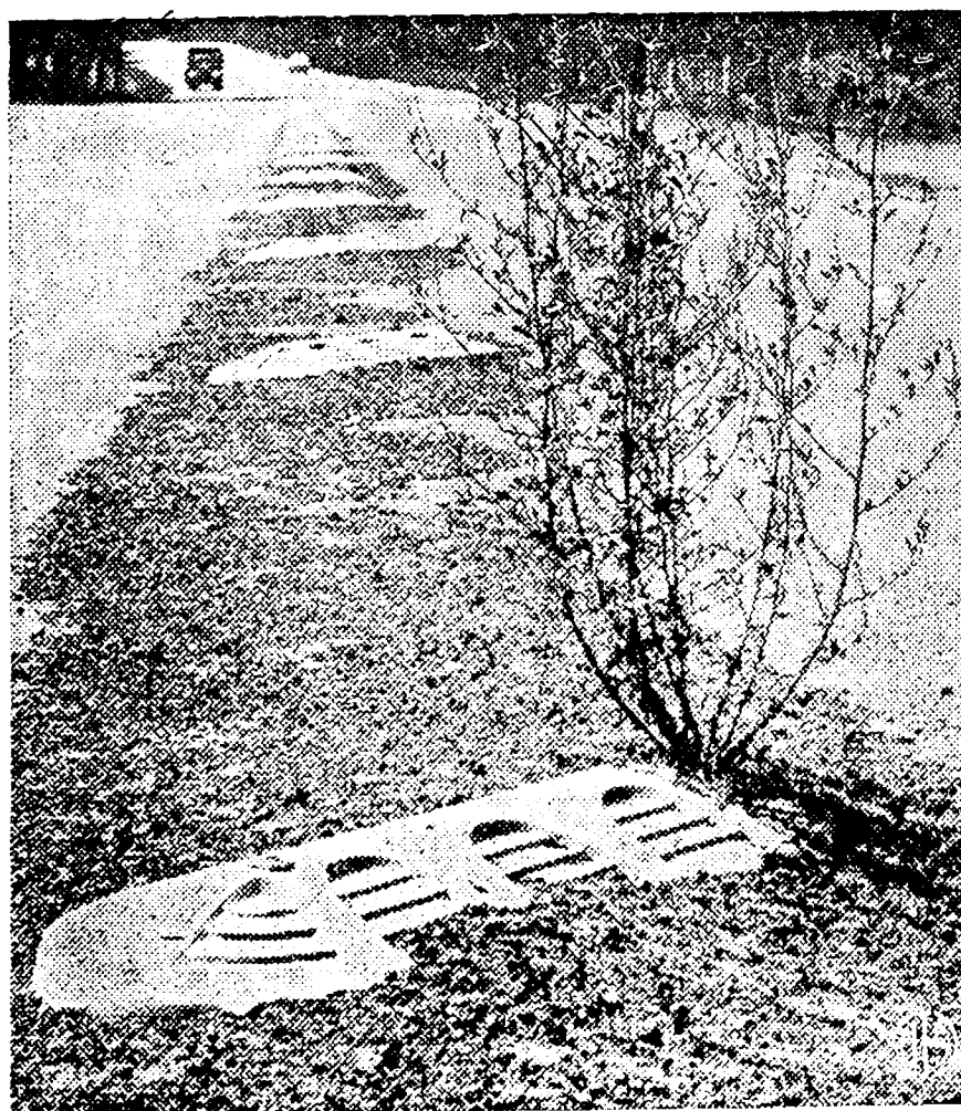
ROAD OF LIFE —Thrusting up through concrete and macadam, this weed clings to life on U.S. Route 220, just west of Williamsport, Pa. The plant is thriving despite its rocky bed and the menace of speeding cars on the four-lane highway.
