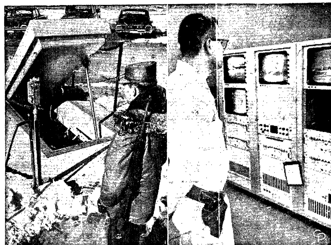
The entrance is a hydraulically-operated door, guarded by Airman 2/c Frank Law- head of Jacksonville, Fla., plus television. Capt. David Cowan, Rochester, Mich., watch- es entrance via television. TV also scans control panels and potential danger points.
