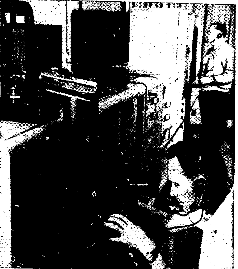
MOON PHOTO RECEIVER —This is NASA's Jet Propulsion Laboratory Deep Space Instrumentation and Film Recording System at Goldstone, Calif., for receiving Moon photos televised by Ranger 8. A technician (foreground) checks the cathode ray tube for viewing Ranger 8 signals and another (background) monitors the video tube for capturing the entire sequence of lunar photos. Camera (upper left) is for recording all photos on 35-mm. film, and Polaroid camera mounted atop the cathode tube is for taking pictures at random for technicians to check quality.
