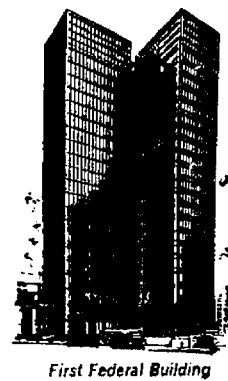
First Federal Building
