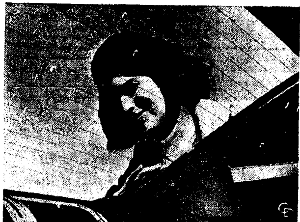
WINDOW DEFROSTER —This auto window defrosting device—narrow strips of a ceramic-metal mixture developed by PPG Industries in Pittsburgh—is set as optional rear window equipment for some 1969 autos. It defrosts electrically.
