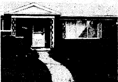
AVON COURT Vacant for over 2 years. Water in back yard pool stagnant for 2 years.
