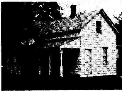
VERNIER ROAD Condemned for over 2 years
