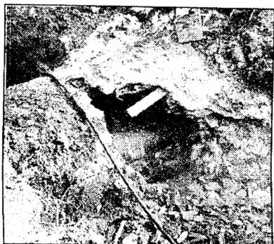
The plastic pipeline can be seen here through a hole in the existing sewer on the north side of Lakeland.
