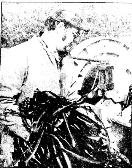
Here Baily gathers shreds of plastic that have been sheared off the thick plastic tubing to make both sides of the joint fit flush together.
