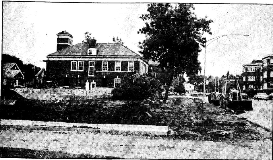
Above: A view of the northwest side of the old fire station. The foundation for the apparatus bay addition can be seen, and the mound of dirt next to the curb in the foreground will be a grassy median. Cars will be able to enter the expanded parking lot through a driveway (foreground) from Maryland (at right).
