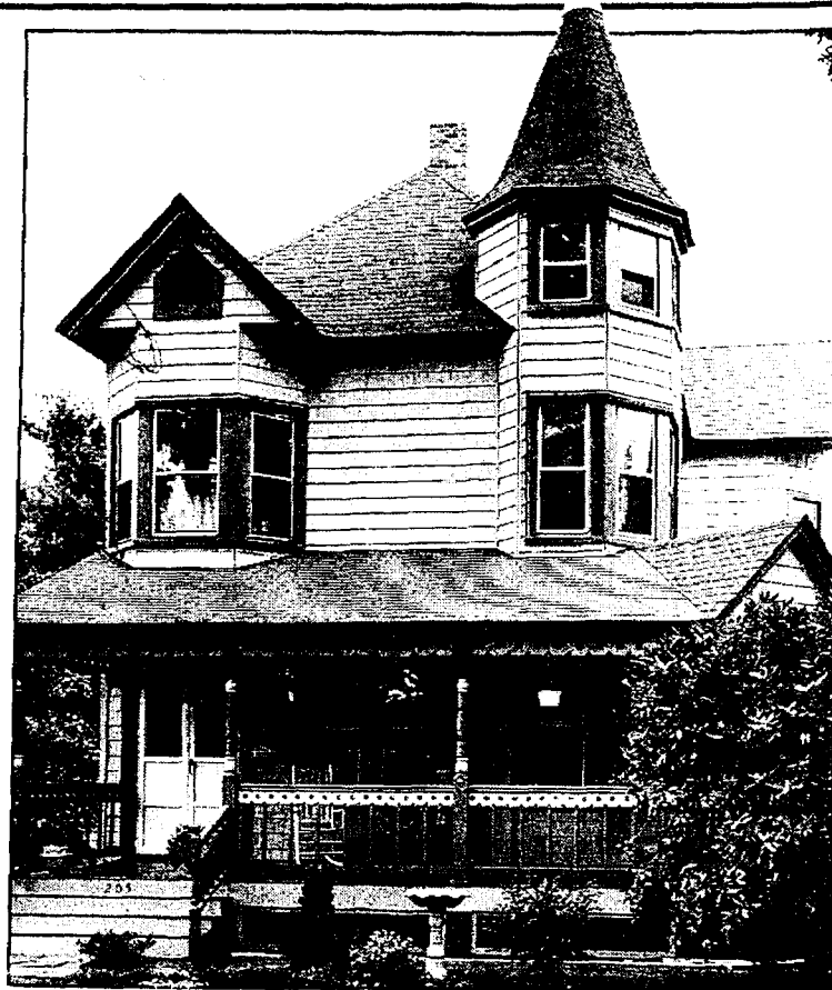
THE SIDING used on this Victorian-style home is remarkably faithful to the texture and dimensionality of hand-split cedar shingles. CertainTeed Corporation's Cedar Impressions™ is manufactured in molds patterned after real cedar shingles.
