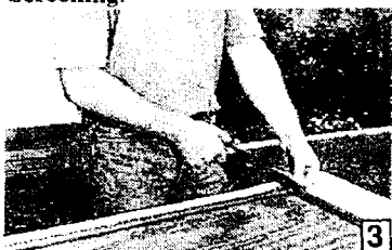
3 ALLOW ALUMINUM SCREENING to overlap spline groove approximately 1/2-inch and cut beginning corner at 45-degree angle.
