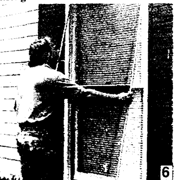
6 TRIM SPLINE END and you have a good-looking screen ready to protect you and your family from summer pests.
