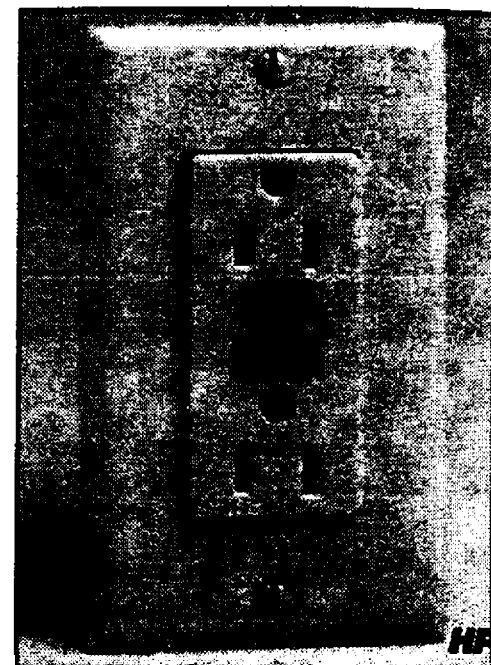
Ground-fault circuit interrupters, which most codes require for electrical outlets installed in kitchens, baths, laundry rooms and garages, automatically shut off power to the circuit on which they're installed when their built-in sensors detect a shock hazard.
