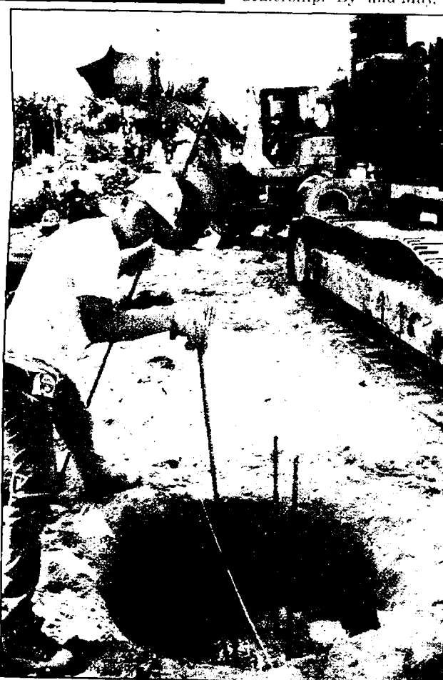
Photos by Brad Lindberg Above left, James Noland of S.L. Shekell construction, watches Ron Howard crawl inside the framework of what will become a 72-ton, steel-reinforced concrete slab to support a section of the new Grosse Pointe Park branch library over a large underground drainage tunnel. The building's foundation will be anchored on cement caissons built by employees of Rohrscheib Sons Caissons, including Aaron Croo, left.
