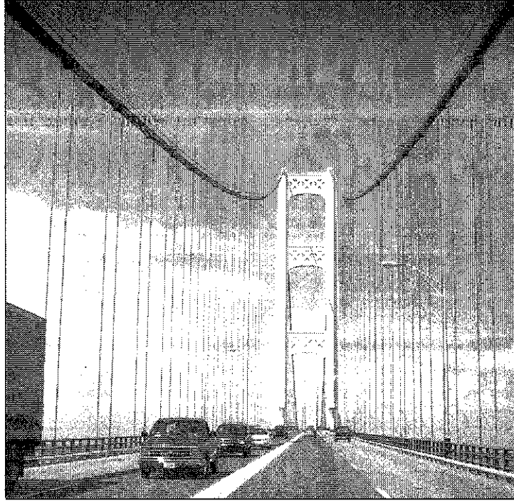
Two towers of the Mackinac Bridge rise 552 feet above the water. The bridge is maintained by a crew of 50, painting, removing snow, repairing the concrete and metal parts of the 50-year-old bridge.
