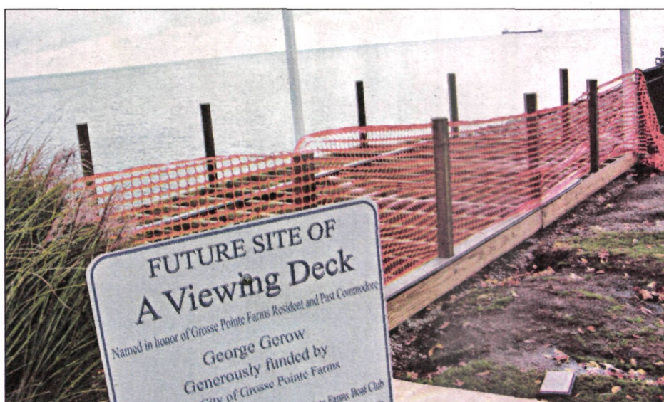
Deck framing is almost ready for planking at a lakeside observation platform being constructed at Pier Park.
