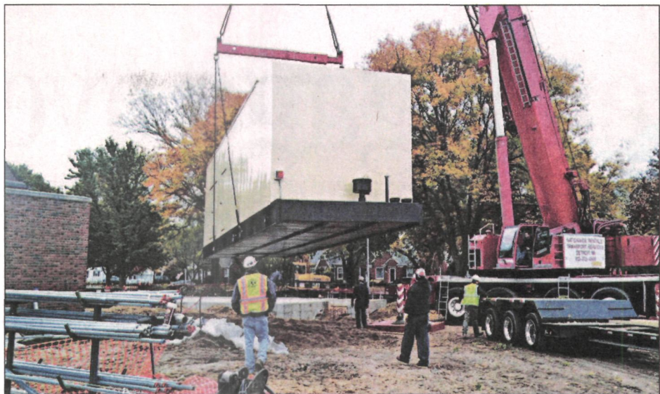
PHOTO BY ADAM GOHS The 77,000-pound permanent generator at Kerby Pump Station is lowered onto a foundation four-feet thick.
