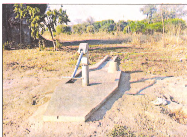
A newly installed water pump.
