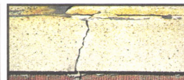
Chimney with cracked cap
