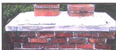
Improperly Designed Chimney Cap
