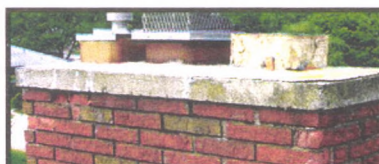
Chimney with cap damage
