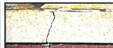
Chimney with cracked cap
