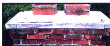
Improperly Designed Chimney Cap
