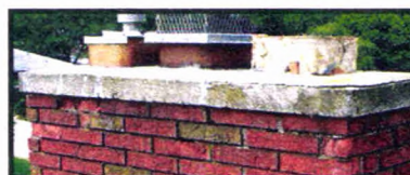
Chimney with cap damage
