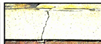
Chimney with cracked cap
