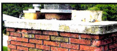
Chimney with cap damage
