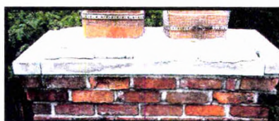
Improperly Designed Chimney Cap
