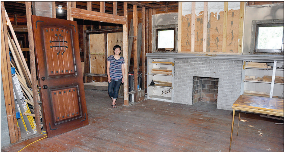
Victoria Li stands near the doorway to the front room. Propped against the studs is a door that was donated.
