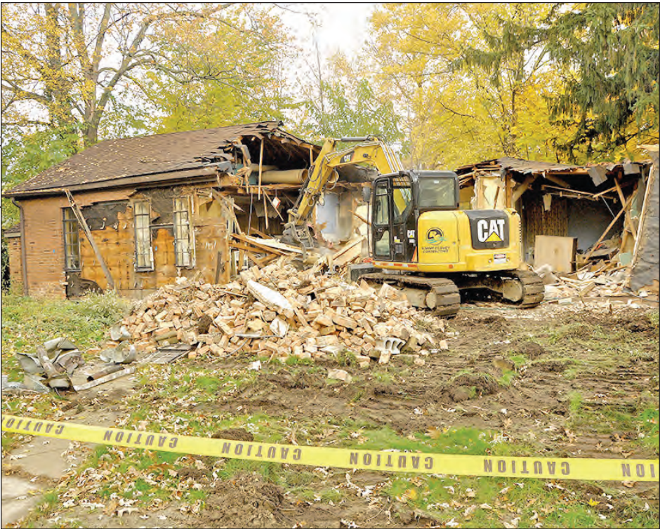
A house on Hawthorne was torn down in November.
