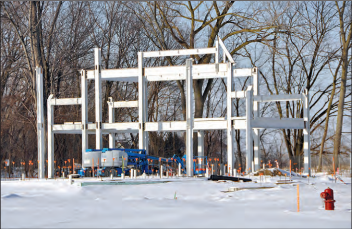
The bones of the new administration building have been erected. Set to open in spring 2020, the buildings will offer opportunities to view permanent, changing and community exhibits; a space for youth educational and adult learning programs; a second-story setting with lake views for corporate and private social events or meetings; a restaurant with indoor and outdoor dining options for lunch and dinner; and an expanded retail destination with merchandise unavailable elsewhere locally.
