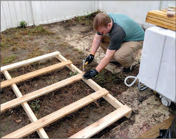
Aaron Beckius constructs a garden box for the Howard family.
