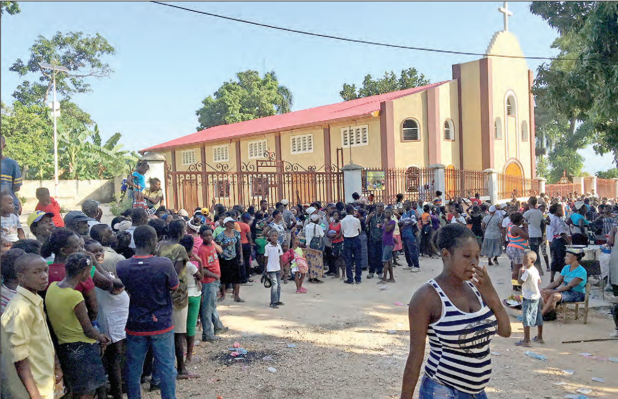
HART built St. Jude Church. “We spent a couple years back and forth to Haiti overseeing construction of the church,” Petz said.
