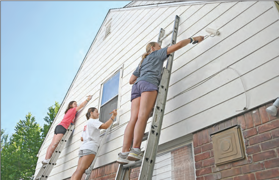
Sydney Hottovy, Cadence Whited and Chloe Dirks touch up the paint on the siding at 1745 Roslyn.
