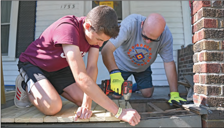
Matt Cassidy and Will Huber put new boards over the hole in the front porch of 1753 Roslyn.
