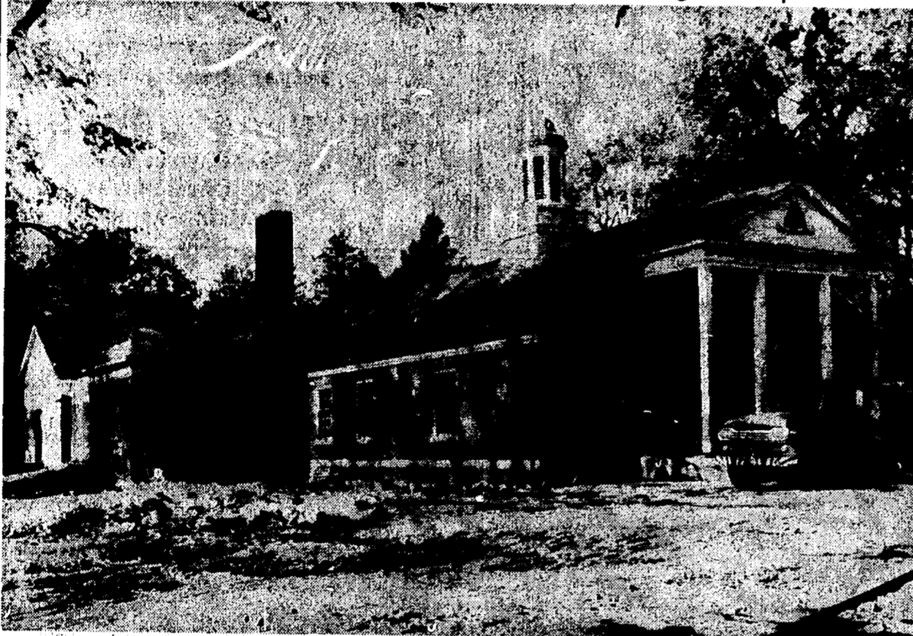
Although about a month behind schedule, the new municipal building in Grosse Pointe Woods, is expected to be completed about the middle of November. Dedication ceremonies have been scheduled for December 2.
