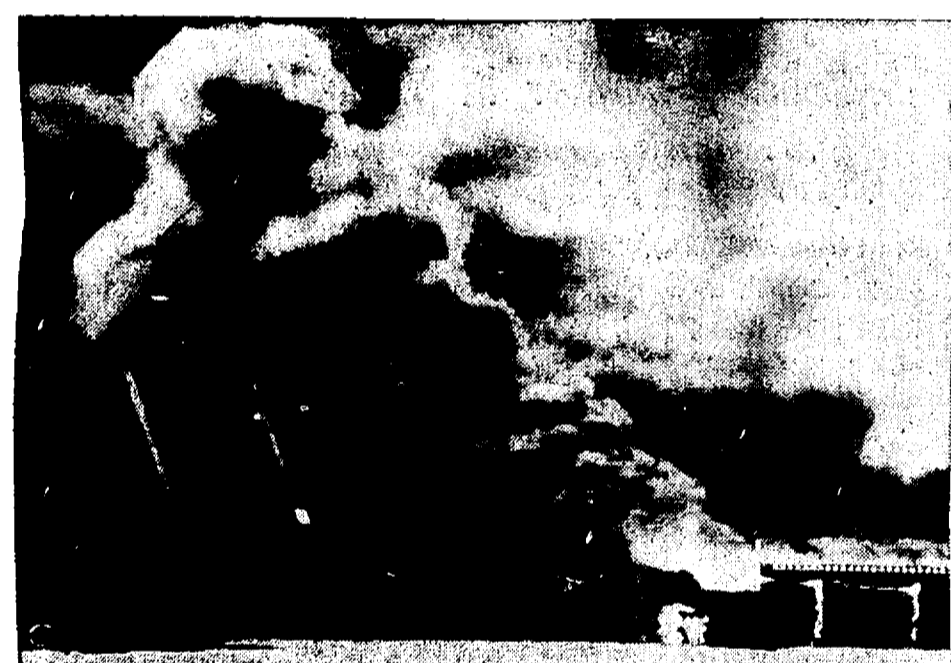
FIRE WRECKS RAILROAD BRIDGE —About 100 feet of the Chicago & Northwestern Railway bridge across the Fox river in Green Bay, Wis., was destroyed by a fire of undetermined origin. Traffic over the bridge was re-routed to the Milwaukee Road tracks.
