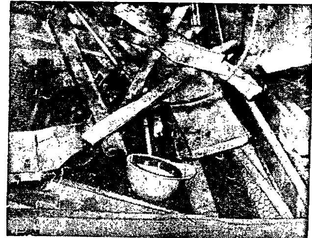
DEATH PLUNGE SCENE —A crash helmet of one of three carpenters killed in a 46-story plunge in Chicago lies in debris of a scaffold which broke. The accident occurred inside a spire of naked concrete, the east core of a twin, circular-shaped skyscraper going north of the Loop. Victims were Homer Fields, 33, James R. Toner, 24, and Wallace Kumpula, 42. They were working on the scaffold.
