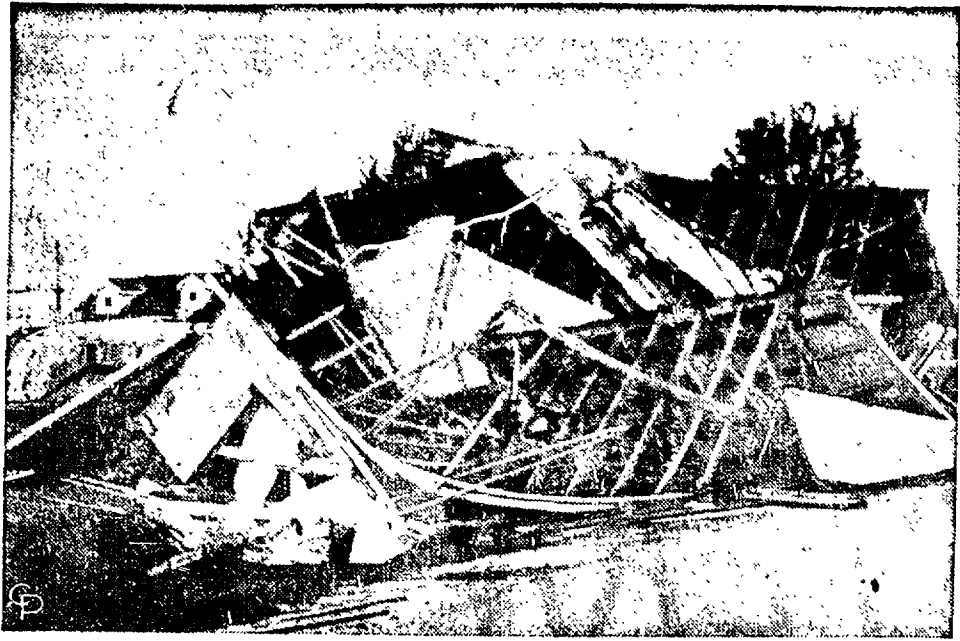
TORNADO FLATTENS CONVENT —A tornado stirred up by Hurricane Carla demolished this convent in Kaplan, La. No one was killed.
