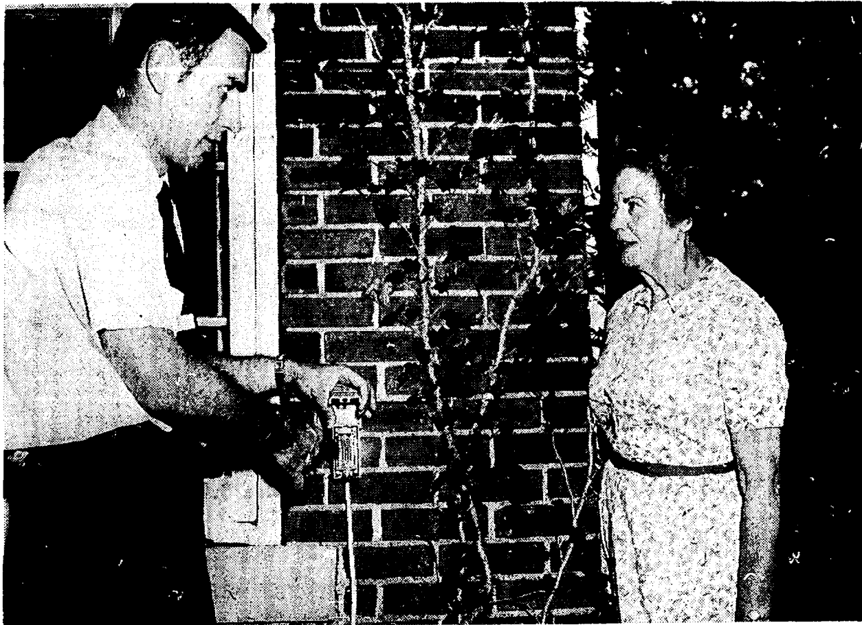
City of Grosse Pointe's Director of Finance, ROBERT C. BENDZINSKI, was on hand when the City installed the first new remote unit for reading water meters at the Washington road residence of Mrs. Sidney M. Caldwell. This makes it possible for the meter reader to get a reading without entering the house.
