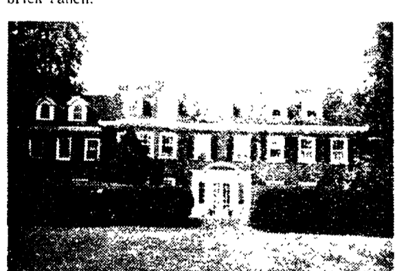
ESTATE WITH ELEGANCE — Excellent condition for the discerning couple. garage apartment. Over $500,000.
