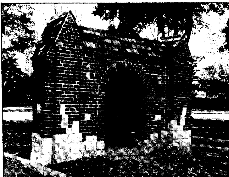
The structure at Oxford and Lakeshore in the Shores has undergone major structural renovations this summer. The Grosse Pointe Historical Society has donated $2,000 to help complete the work.
