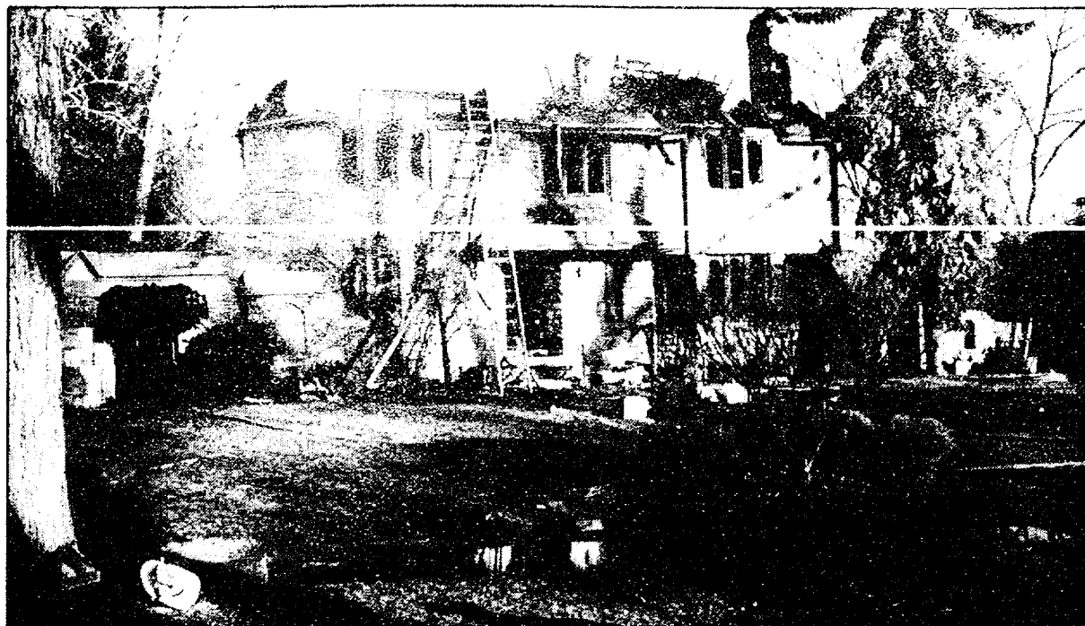
Fire gutted the Schroeder residence on Lakepointe in the Park early Dec. 13. The family escaped after their smoke alarm sounded.
