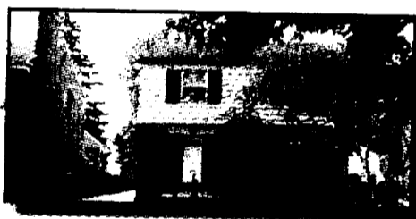
GROSSE POINTE WOODS $210,000 CLASSIC BRICK COLONIAL. Large family room, 19x14.6 with natural fireplace, newer two and one half car garage, many newer windows, walk-up attic, central air, six panel doors. Immediate occupancy. (GPN-H-41VAN) (313) 885-2000
