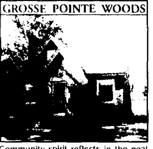
GROSSE POINTE WOODS Community spirit reflects in the neat homes surrounding this charming all brick bungalow. Living room and family room each feature a fireplace. Many updates throughout: roof, windows, furnace, central air and side doors. $244,700 SC17ROS 586-778-8100
