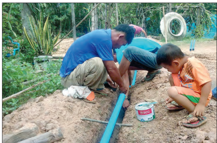
Villagers lay water pipes.
