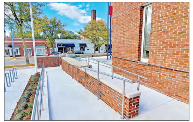
A new ramp complies with the Americans with Disabilities Act.
