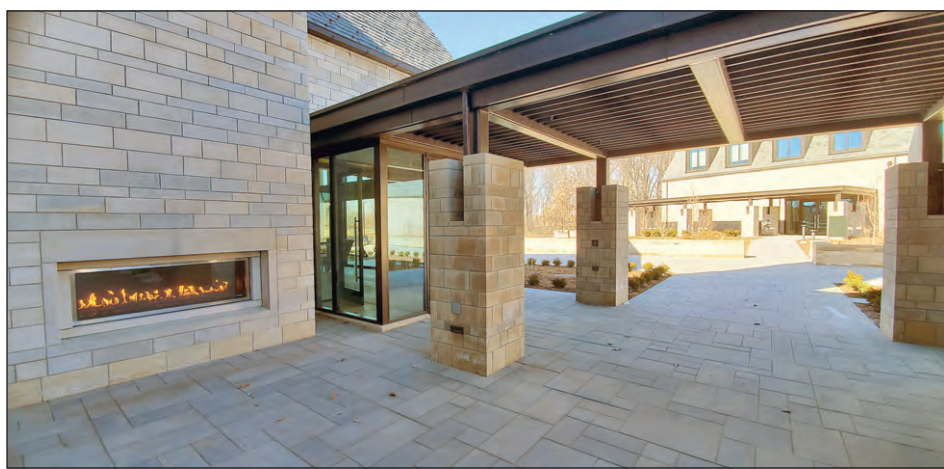
The outdoor fireplace on the patio of the visitor center.
