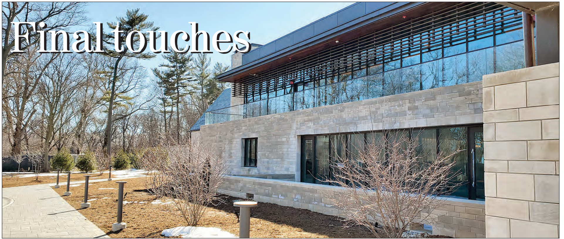
A view of the restaurant patio on the first floor and the larger event space on the second floor with a balcony. The bird-safe glass prevents bird casualties caused by heavily windowed buildings.
