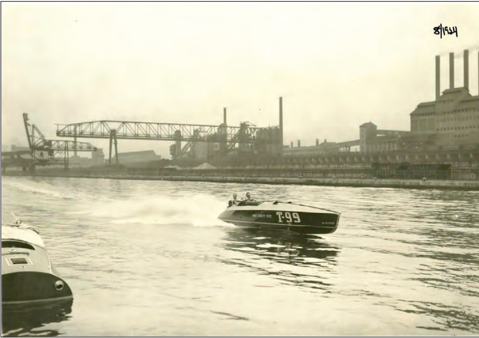
Edsel Ford modified airplane engines leftover after World War I for use in powerboats.
