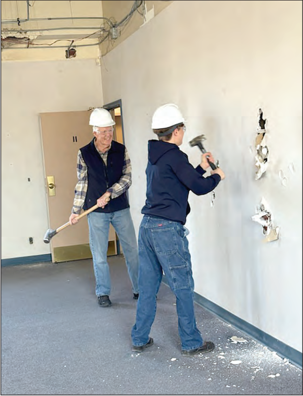
Gary and Stephen Van Elslander participate in the demolition of the future store. Gary Van Elslander is on the Full Circle Board of Directors.
