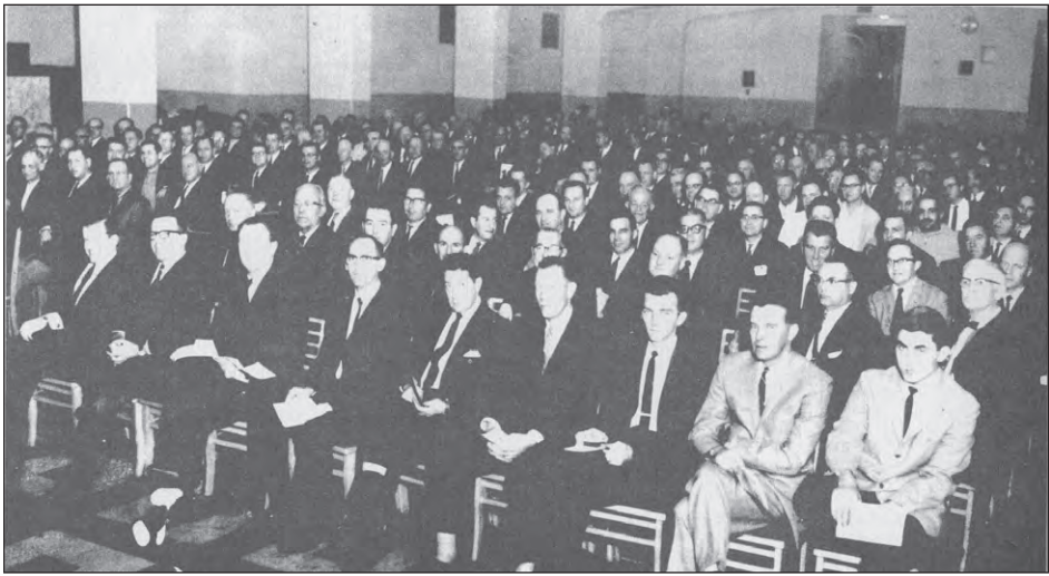
Left, St. Clare parishioners fill council chambers in 1963, when they requested a permit for a new school building, as well as the closure of a portion of Audubon. Right, Cardinal Edward Mooney lays the cornerstone of the new church.
